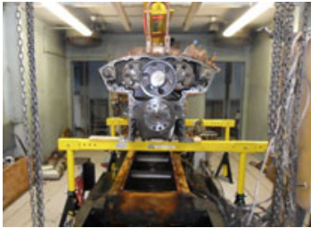
Source: Wessex Water Plc
