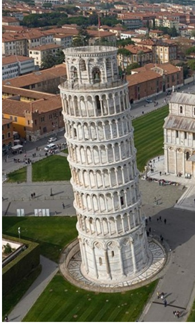
Figure 2: The Leaning Tower of Pisa went sideways because its builders didn't understand that the ground below one side was softer than the other [6]
