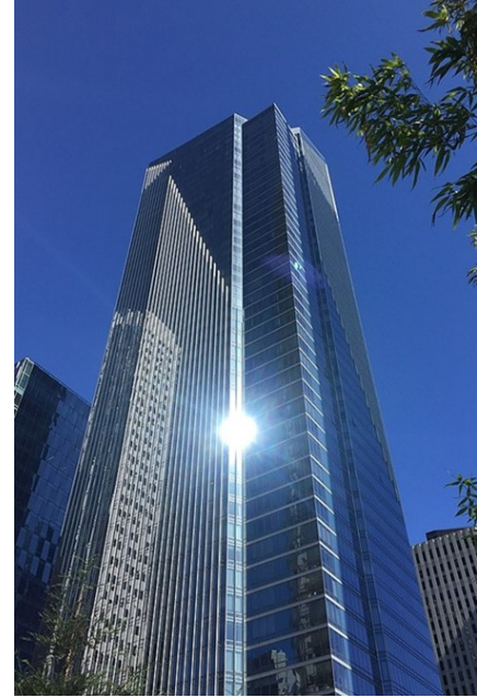
Figure 4: San Francisco's Millennium Tower [8]
