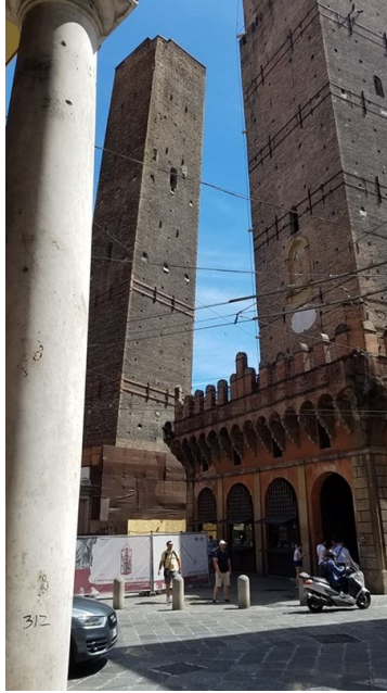
Figure 3: The Bologna Leaning Towers [7]
